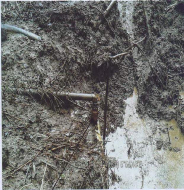
4" Valve connected to 3" pipe installed by vandals for the purpose of oil theft.
