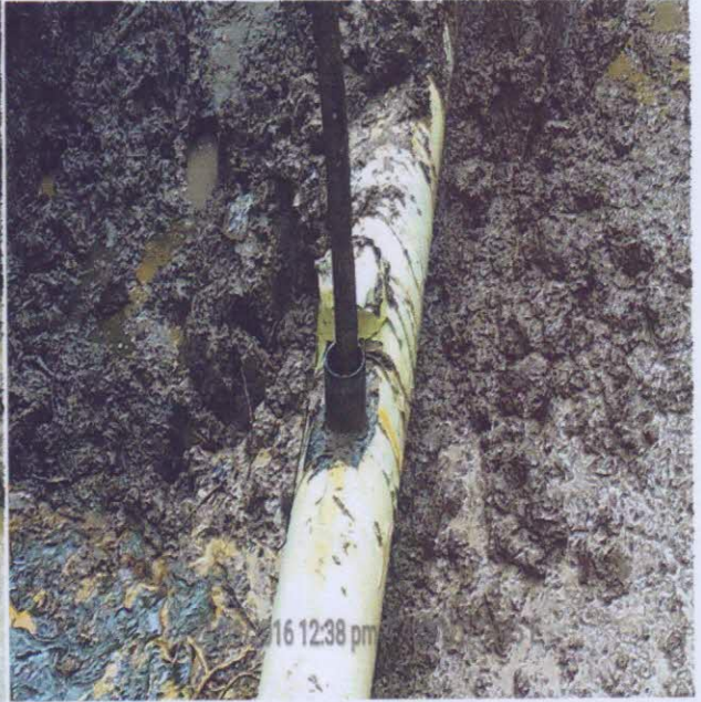
4" Valve connected to 3" pipe installed by vandals for the purpose of oil theft.
